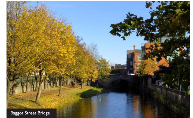
Baggot Street Bridge
